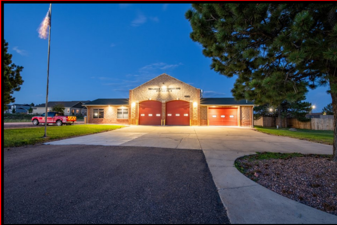
Fire Station 3 1855 Woodmoor Drive Monument, CO 80132
