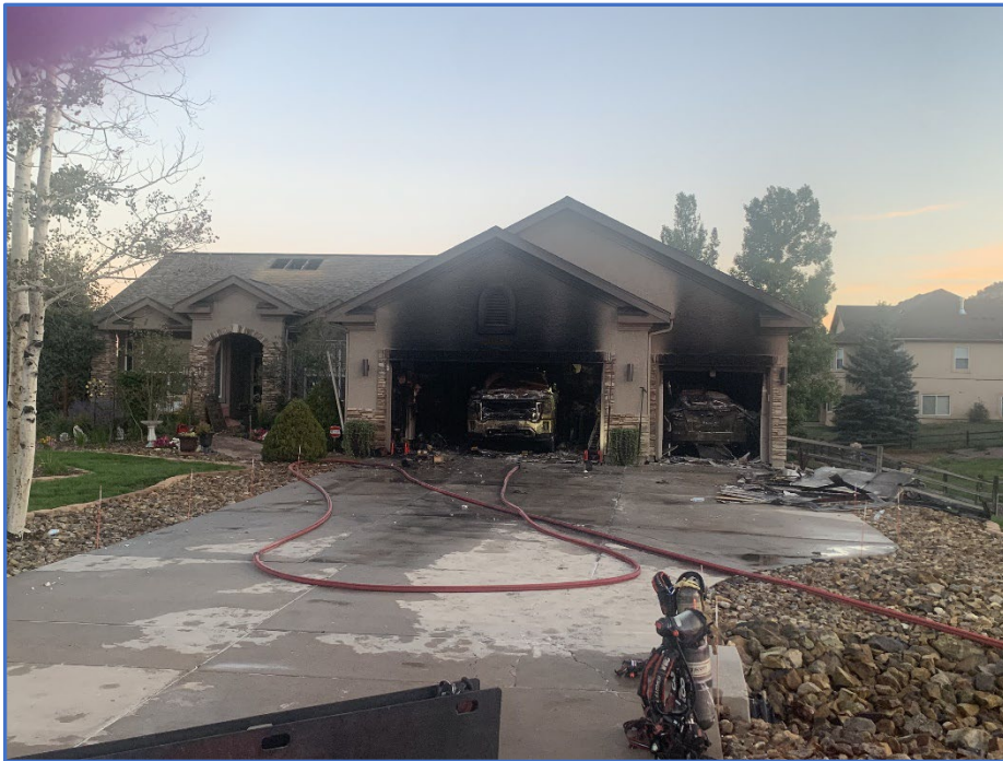
Structure Fire on True Vista Circle.
