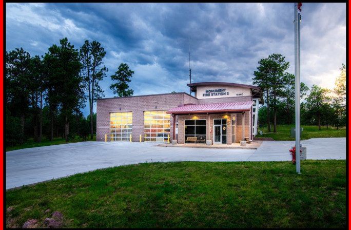
Fire Station 2 18460 Roller Coaster Road Monument, CO 80132
