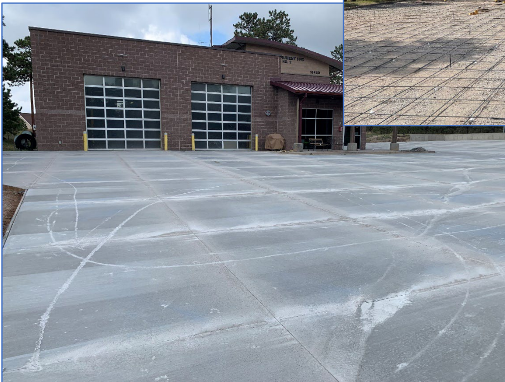
New concrete apron at Fire Station 2
