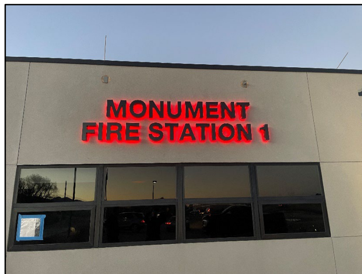
Monument Fire Station 1 signage
