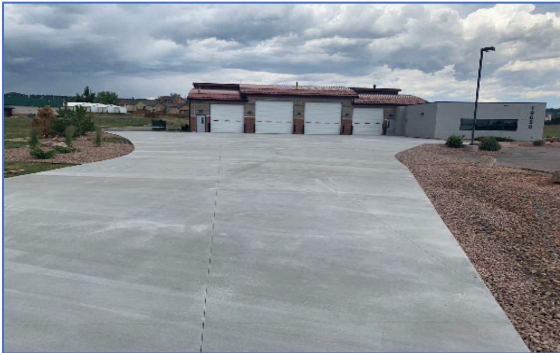
Fire Station 1 concrete apron.
